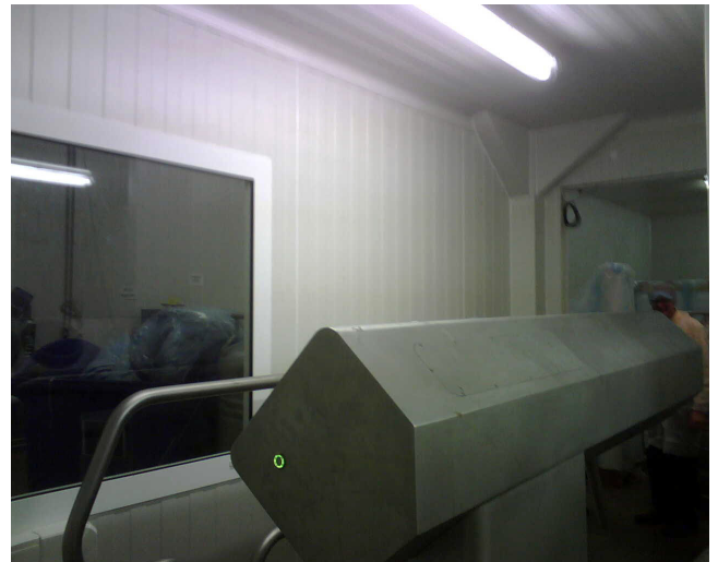
Interlock buffer between not classified and classified area with shoes and hands washing
