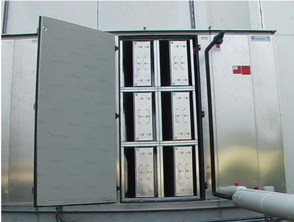
Automatically sanitised air treatment unit equipped with electrostatic filters and ionisers installed in a large food processing plant of a multinational company in Northern Europe.
