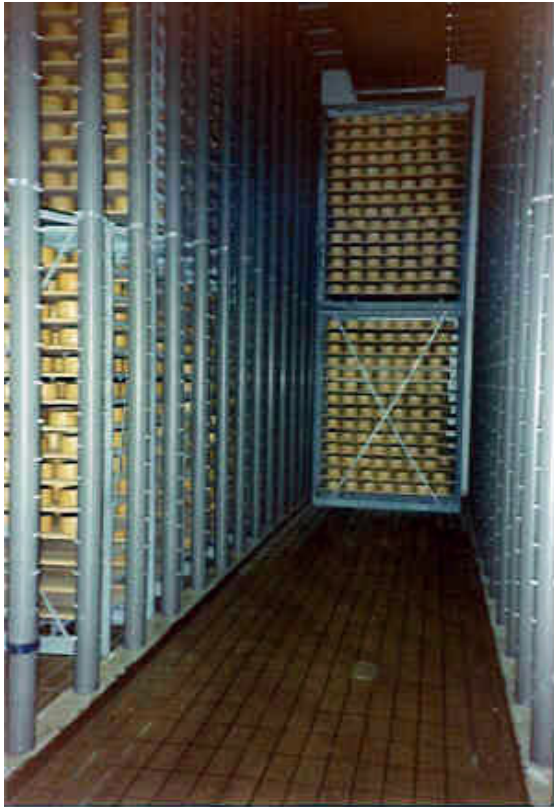
Storage system for racks with deep diffusion air distribution.
