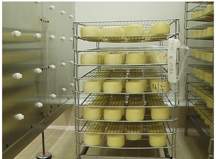
Cheese ripening system with deep air diffusion and contamination control.
