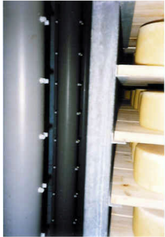
Air distribution nozzles, to allow the air flow to gently surround the product.
