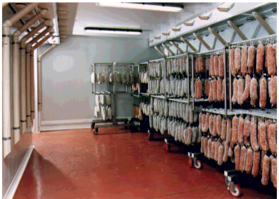
Drying room for sausages with special swinging air distribution system.
