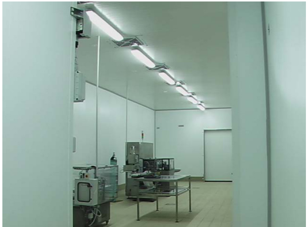
Clean Room for packaging Class 10,000 according to FS 209E with AirClean system
