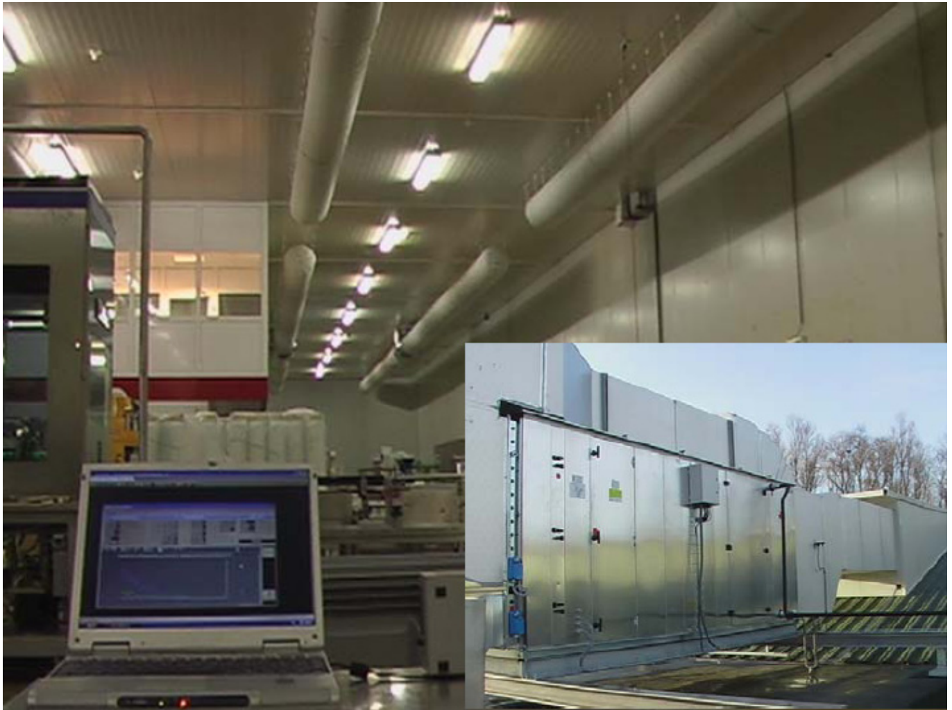
Contamination controlled room ISO 7 through AirClean System
