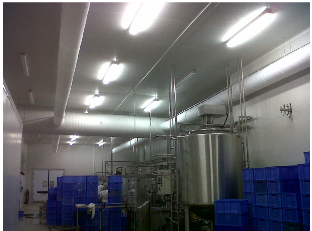
Gulgun dairy factory in Nicosia (Northern Cyprus) under construction.
